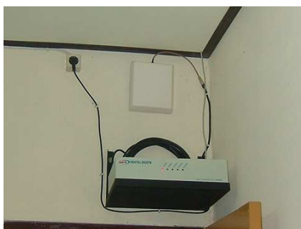
7 dBi GSM board antenna
